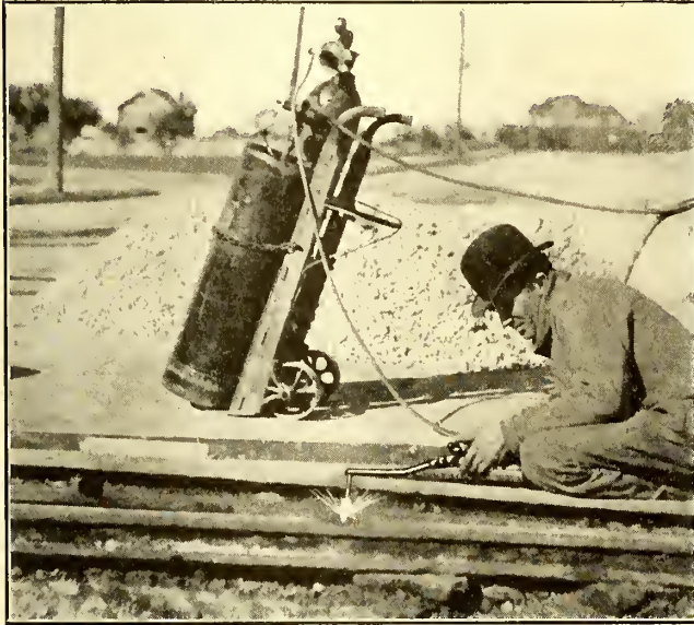
GAS-CUTTING OUTFIT MOUNTED FOR WORK IN THE STORAGE YARD
